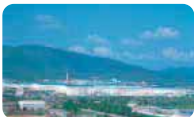
LG Air Conditioning Division, Korea
